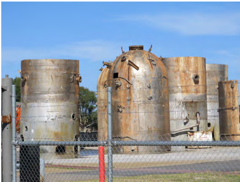
Figure 4. Parts of the deconstructed Tantanoola pulp mill. The pulp mill was shut down in December 2010 (Authors).
